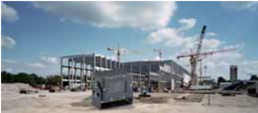
Construction machinery and cranes
